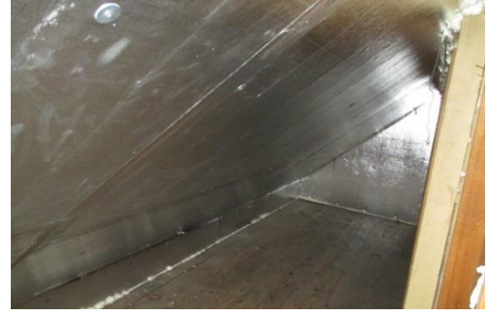
Method B, using foil-faced polyiso foam board as vapor barrier and air barrier.
