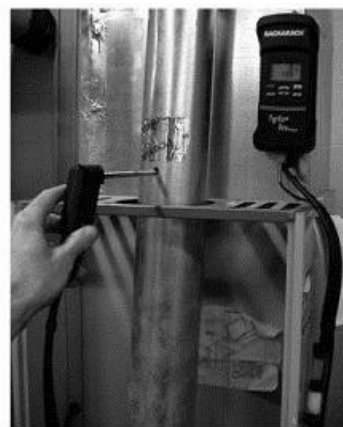
Testing 80+ furnaces: Drill a quarter-inch hole in the metal vent connector to sample combustion gases.
