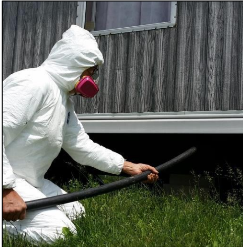
Fill tube inserted into belly hole.
