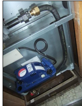
Condensate pumps: These small pumps install in the furnace cabinet.
