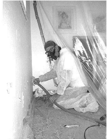
Wall-blowing tent: This tent protects the customer and their belongings from insulation and paint dust.
