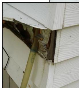
Bowing walls: Using a fill tube works well for most mobile home wall cavities.
