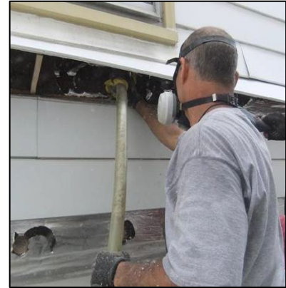
Tube-filling walls: Insulation is dense-packed into walls using a fill tube inserted into the wall cavity.
