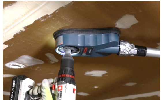
Lead-safe drilling: Using a shrouded drill with a HEPA vacuum removes dust where it is generated.
