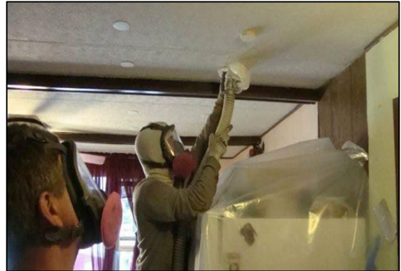
Installing insulation through the ceiling: The technician pushes the fill tube into the cavity and out near the edge of the roof. The holes are drilled in a straight line for aesthetics.
