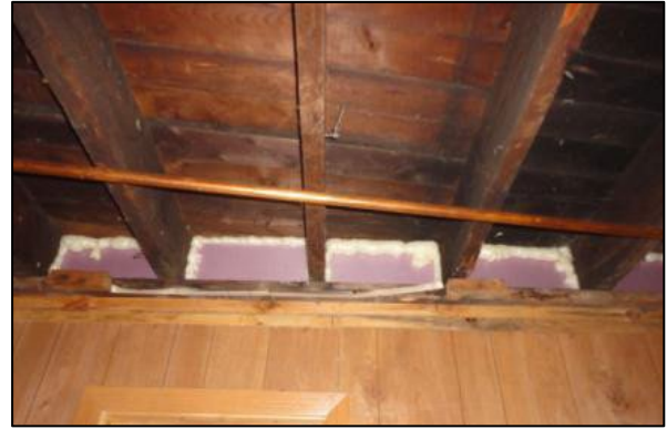
Insulating and air sealing rim joist: Rigid board insulation installed in joist cavities, with spray foam to seal at the edges.
