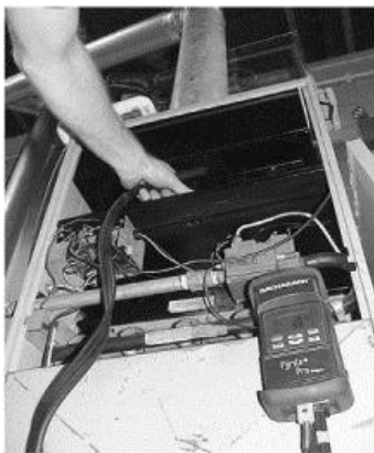
Testing older furnaces: Insert the probe into the draft diverter near the exhaust ports of the heat exchanger.
