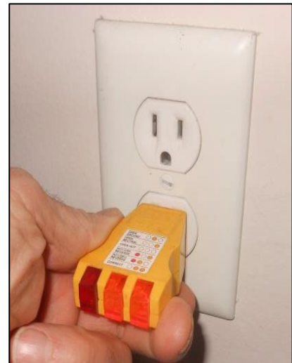
Checking walls: Measure the cavity and the existing insulation level. Make sure wall outlets work before and after insulation installation.
