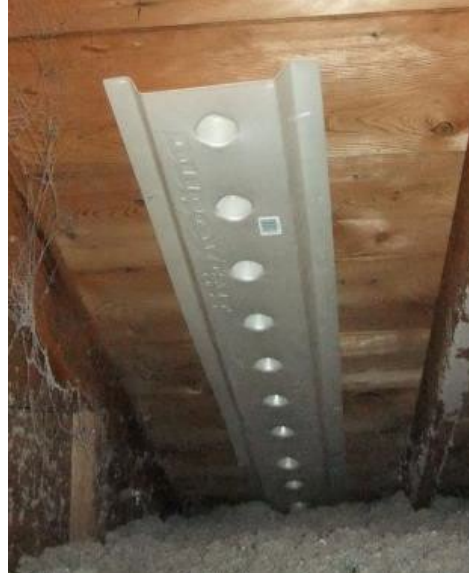
Soffit chute: Allows installation of maximum amount of insulation in this cold area. Also prevents wind washing and airway blockage by blown insulation.
