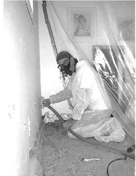
Wall-blowing tent: This tent protects the customer and their belongings from insulation and paint dust.
