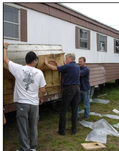
Loosening siding for wall insulation: Remove screws at the bottom of the metal siding. Before installing insulation, fasten the siding sheets together at the bottom with a short sheet-metal screw.
