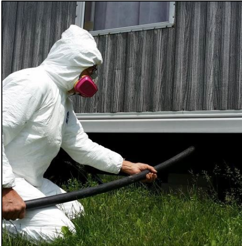
Fill tube inserted into belly hole.
