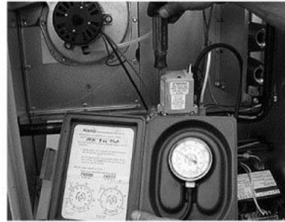
Adjusting gas pressure: Adjusting gas pressure is the only way to change the fuel-air mixture.
