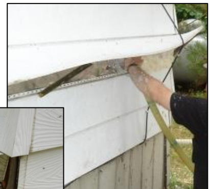
Bowing walls: Using a fill tube works well for most mobile home wall cavities.
