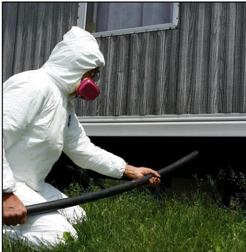
Fill tube inserted into belly hole.
