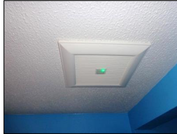
Surface-mounted exhaust fan: Exhaust fans aid air quality by drawing fresh air into the building as they remove indoor pollutants.
