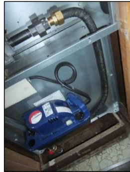
Condensate pumps: These small pumps install in the furnace cabinet.
