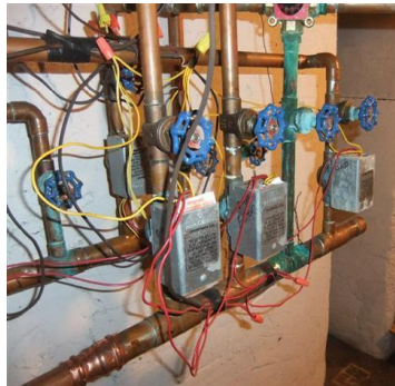
Zone valves: A separate thermostat controls each zone valve. When a thermostat calls for heat, the boiler fires and the zone valve opens.
