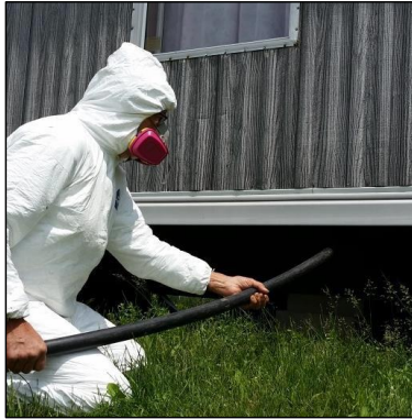
Fill tube inserted into belly hole.
