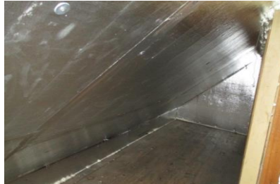
Method B, using foil-faced polyiso foam board as vapor barrier and air barrier.
