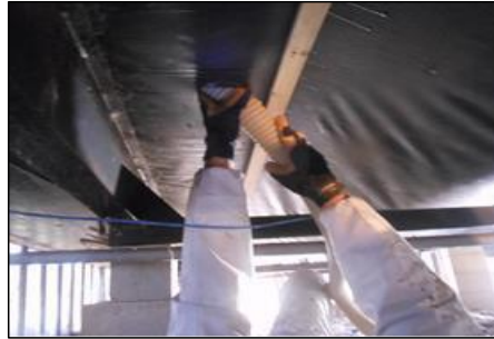
Blowing insulation from under the home: A large diameter fill tube fills cavities rapidly from underneath.
