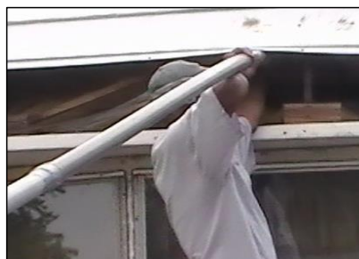
Roof-edge blowing: Use a rigid fill tube to blow insulation through the roof edge. This avoids making holes in the roof, though this process requires much care in refastening and resealing the roof edge.
