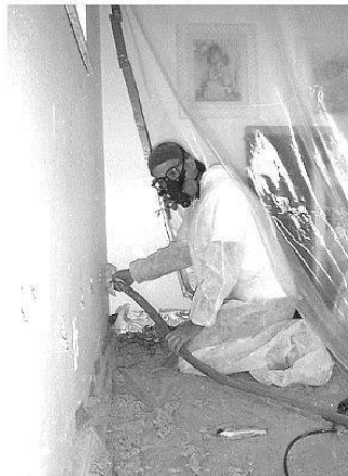
Wall-blowing tent: This tent protects the customer and their belongings from insulation and paint dust.
