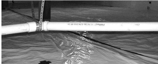
A well-sealed crawl space: The dirt floor in this crawl space is covered with a well-sealed cross-linked polyethylene ground moisture barrier.
