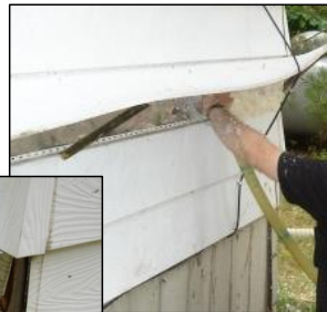
Bowing walls: Using a fill tube works well for most mobile home wall cavities.
