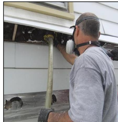
Tube-filling walls: Insulation is dense-packed into walls using a fill tube inserted into the wall cavity.
