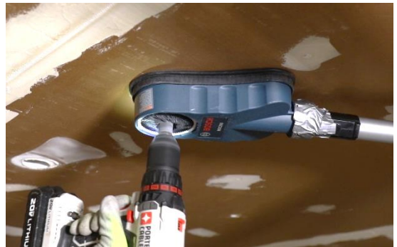
Lead-safe drilling: Using a shrouded drill with a HEPA vacuum removes dust where it is generated.
