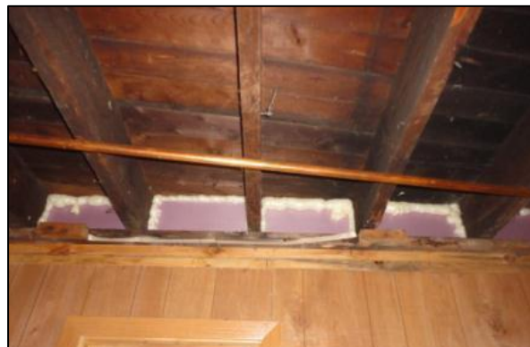
Insulating and air sealing rim joist: Rigid board insulation installed in joist cavities, with spray foam to seal at the edges.
